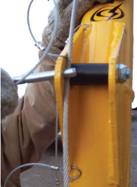
Figure #5.2e: Securing the winch cable to the elbow roller
