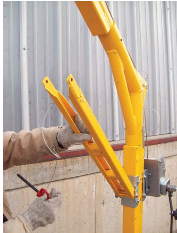
Figure #5.2i: Rotating the elbow support frame into position
