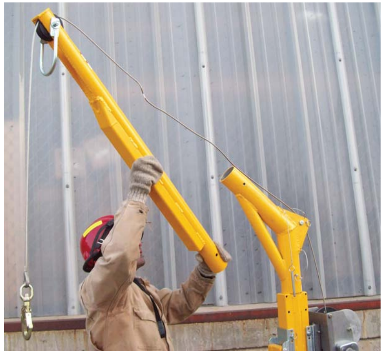
Figure #5.2g: Installation of the offset arm
